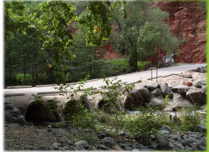
The crossing as seen from the natural beach
